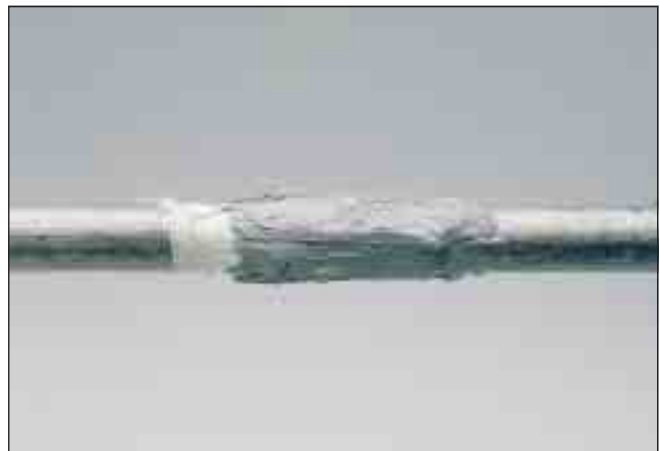
Picture 4 Emergency repair of pipes
